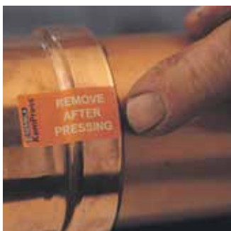
For DN65-100 fittings, remove the KemPress® label to indicate completion of the press.
