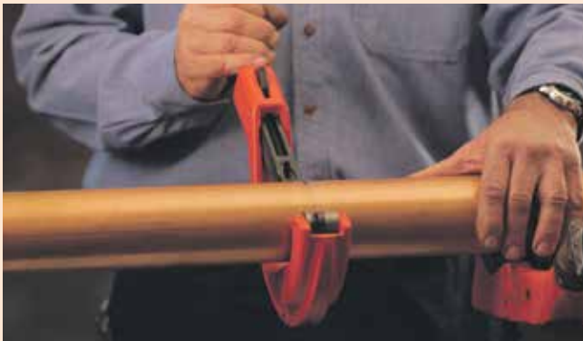
1. Cut copper tube to length using a pipe cutter or fine tooth saw and ensure the pipe is cut square.
