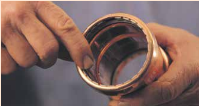
3. Ensure you have the correct sized fitting, check the fitting is clean and the stainless steel grip ring and O-ring are free from debris and correctly seated in the fitting.
