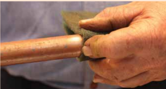
3. For existing copper tube, clean the end with emery paper or a soft scourer.
