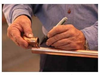
**4.** Mark the insertion depth by lining up the fitting side by side with the tube and mark the tube. When the fitting is inserted onto the tube the outer edge of the fitting must line up with the marking. For correct insertion depths see the table below.
