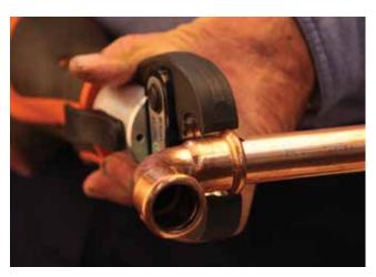
**7.** Check the fitting outer edge still lines up with the marking. Open the pressing jaw and close it around the fitting so the raised bump in the fitting rests inside the groove of the pressing jaw.
