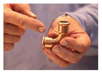
**6.** Check the fitting is clean and the O-ring is free from debris and correctly sitting in place. Push fitting on tube all the way to the engagement marking.
